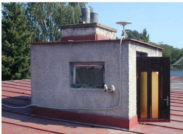
a) Roof of the building
